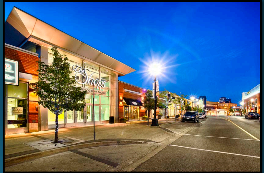
Created new city street
